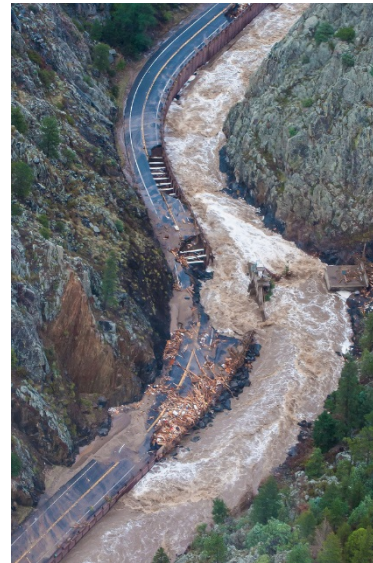
2013: Big Thompson Canyon and washed out US 34 near Estes Park, CO (elevation: ~8000ft) 10 lives lost
