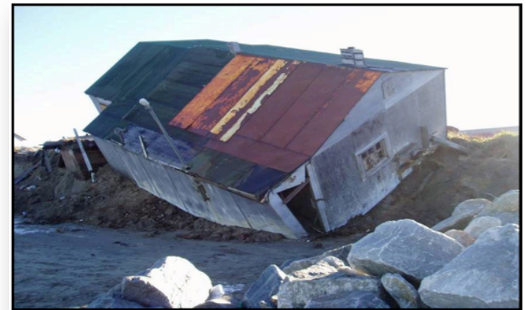
Photo 9: Home falling over eroded bank in Shishmaref. (Credit: Tony Weyiouanna)
